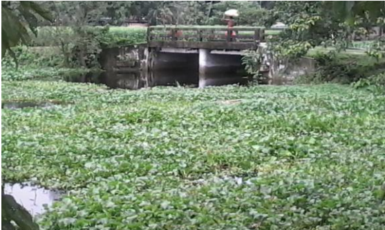
Figure- 10. Reduced channel width due to construction of culvert.
