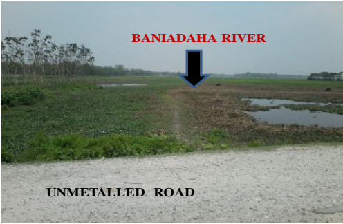
Figure- 8. Construction of road across the river channel at Panishala village.
