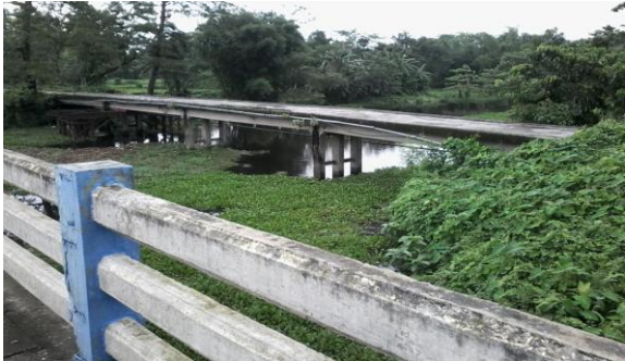
Figure -9. Construction of bridges on river at Ghagir ghat.
